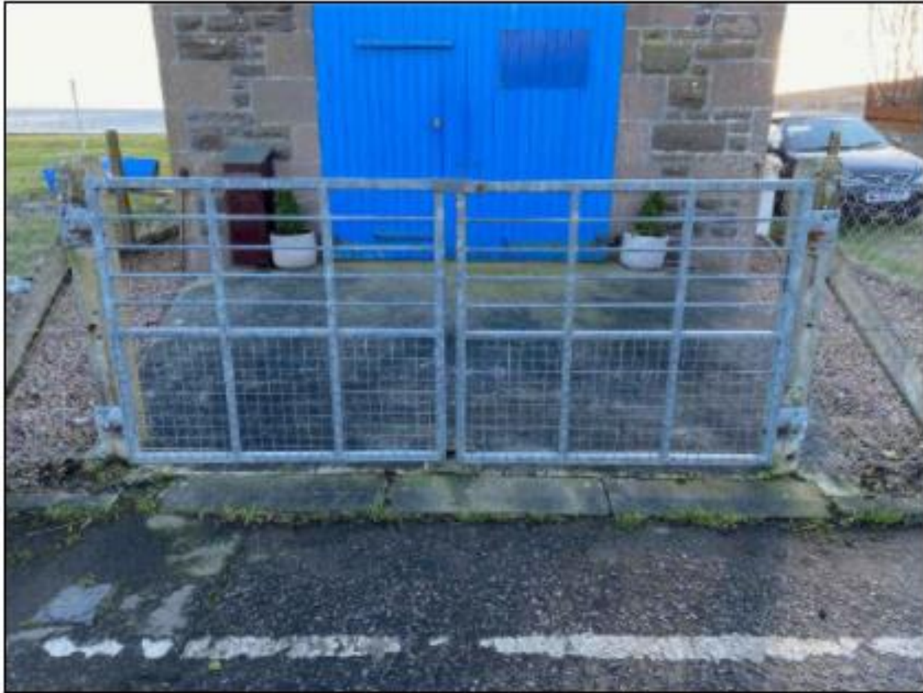
IMAGE OF ENTRANCE - Existing
