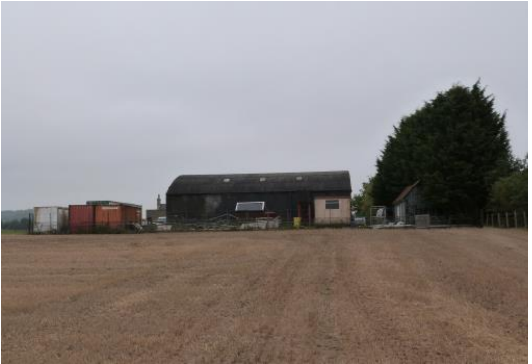
Adjacent buildings and yard
